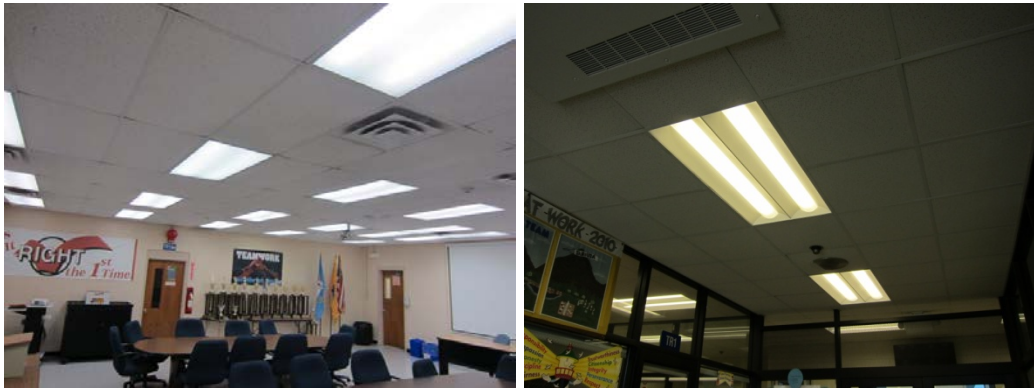
Typical classroom T8 lighting (L); and T5 hallway lighting (R)
