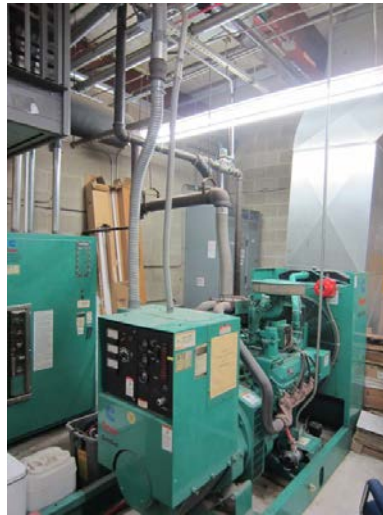
100 kW natural gas generator
