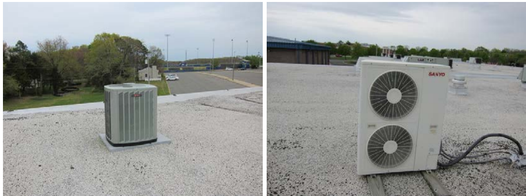
Typical condensing unit for unit ventilators (L) and condensing unit for server equipment (R)
