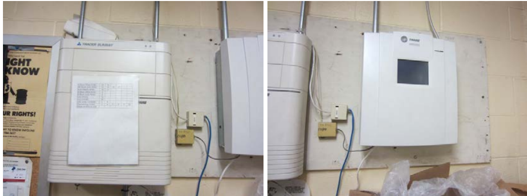
Trane Tracer Summit (L) and Building Control Unit (R)
