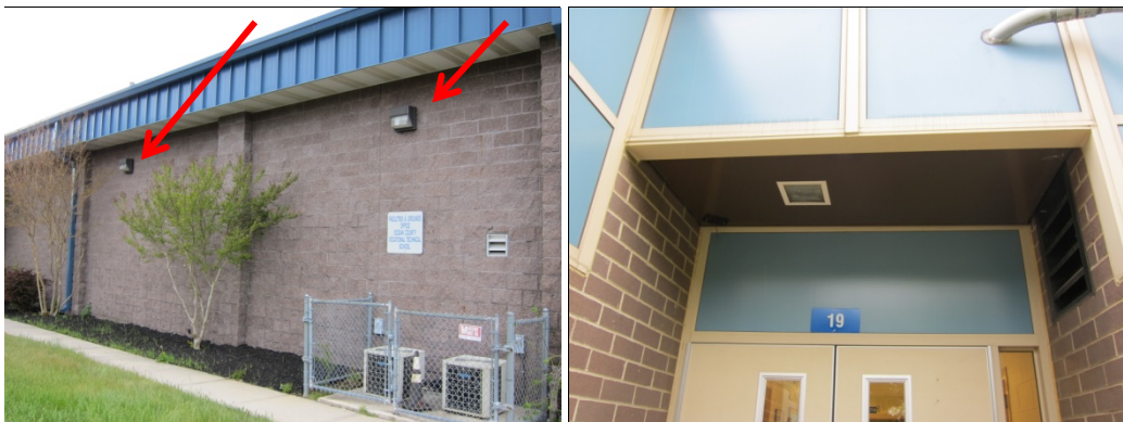
Typical metal halide wallpack fixtures (L) and typical recessed CFL (R)
