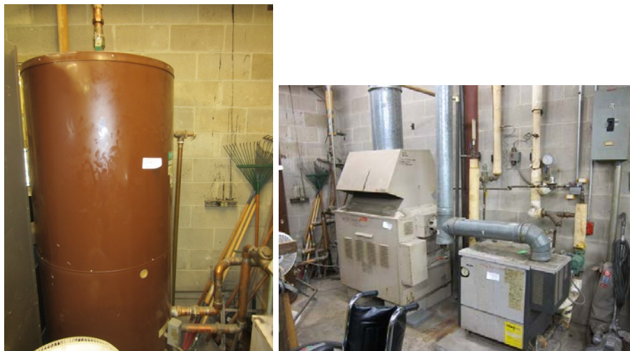
DHW storage tank (L), domestic hot water heater (C) and heating hot water boiler (R)
