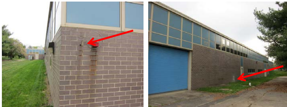
Unsealed wall opening (L) and efflorescence on brick and masonry walls indicate moisture presence within the wall cavity (R)
