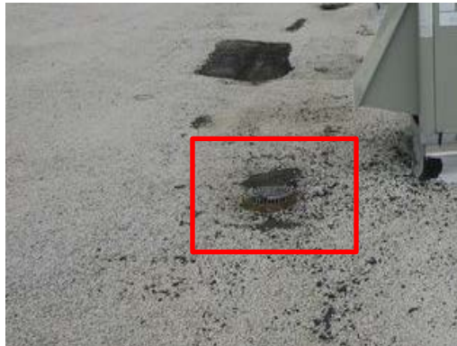
Foliage build-up on roof drain
