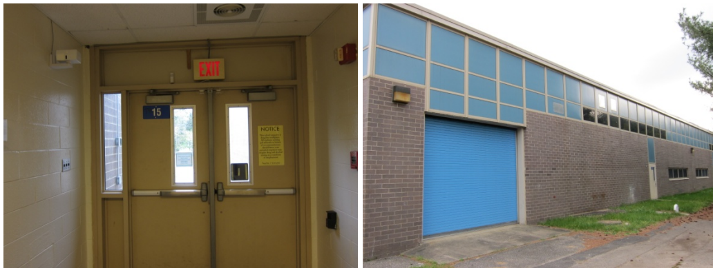
Metal doors with a non-insulated door frame (L) and garage door type (R)
