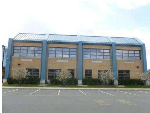
Partial North Façade
