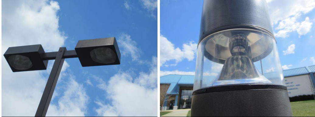
Typical metal halide parking lot fixtures (L) and a typical bollard fixture (R).
