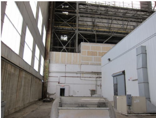
North Façade (inside Hangar 1)
