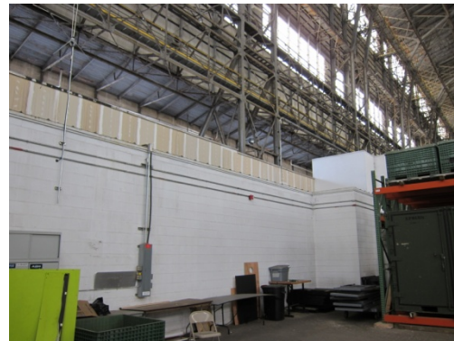
North Façade (inside Hangar 1)
