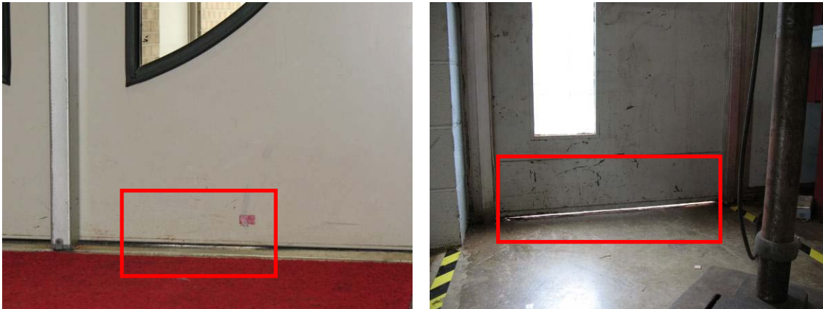
Worn Weather Stripping at Front Door and One of the Shop Side Doors
