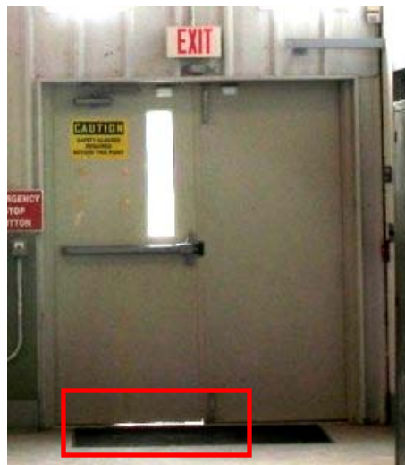
Worn Weather Stripping at Shop Side Door
