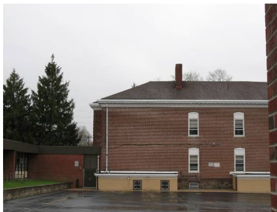
Asphalt shingle roof on older section of school
