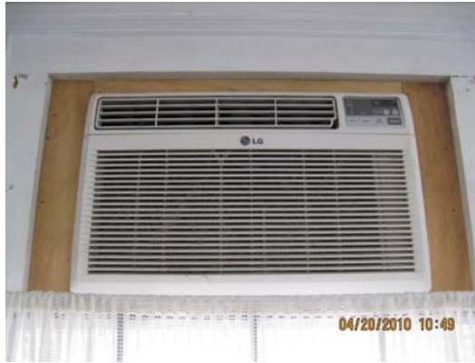
Typical through the window air conditioner found in both offices on the first floor
