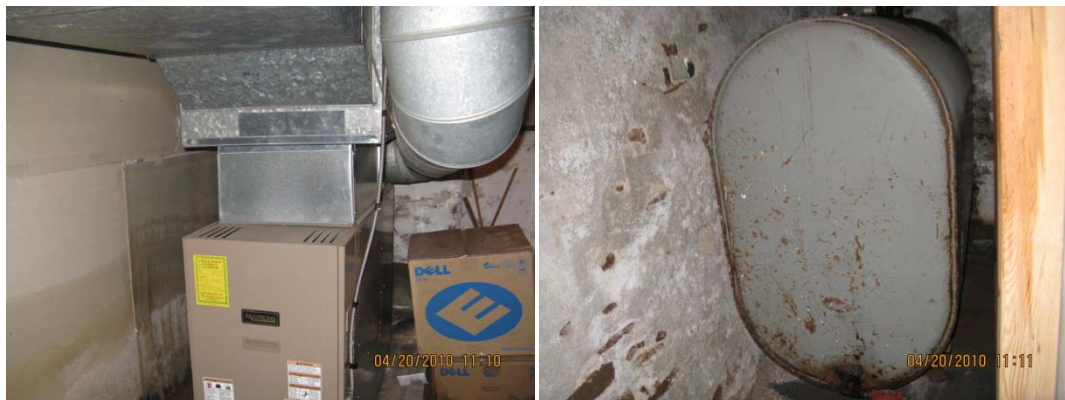
Armstrong Oil Fired Furnace and Oil Storage Tank
