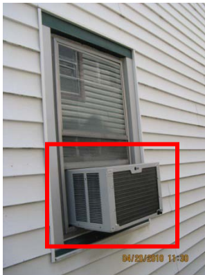
Air-leakage at sleeved window/wall air-conditioning units
