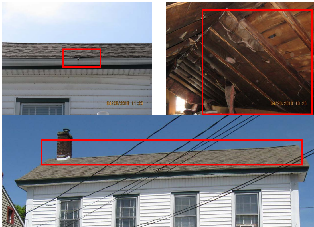
Typical roof system with sections of missing or needing flashing, and signs of displaced shingles and sections of missing, or damaged and ineffective insulation.
