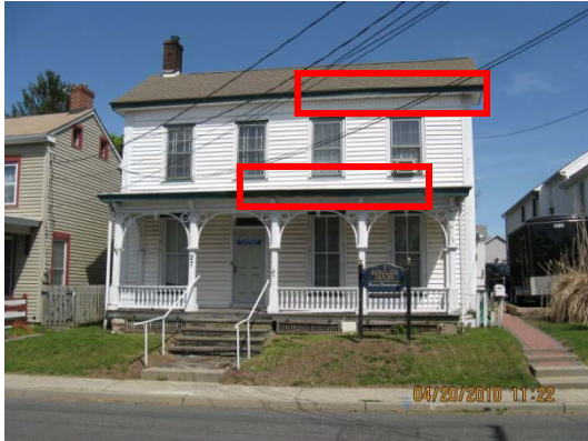
Damaged exterior wall surfaced and signs of water damage from missing flashing and damaged gutters.
