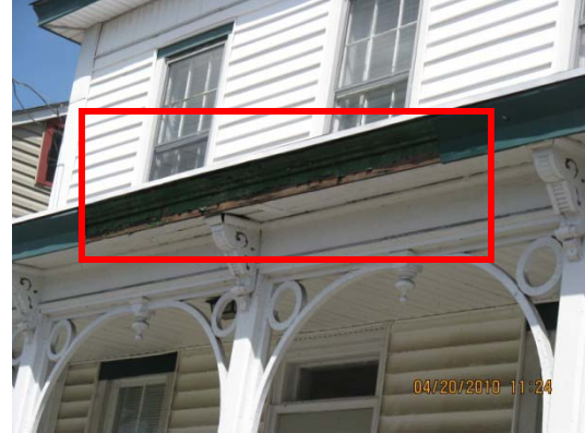
Damaged exterior wall surfaced and signs of water damage from missing flashing and damaged gutters.
