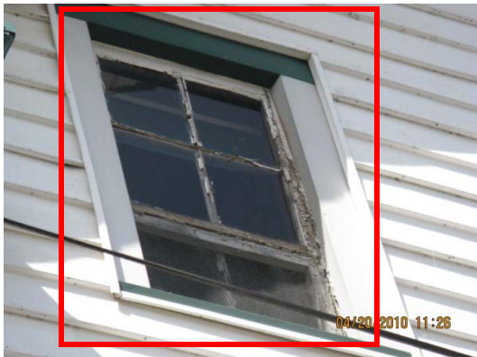
Examples of damaged/aged window frame, and single-glazed window with ineffective frame
