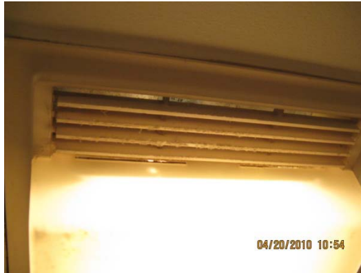
Typical toilet exhaust fan with clogged dusty vents
