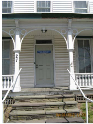
Typical Exterior Door Installations with some sections of damaged or missing weather-stripping
