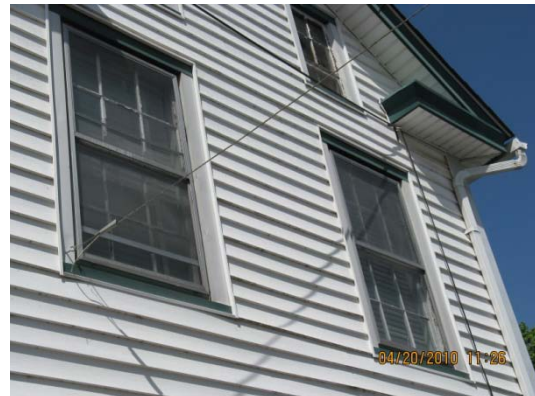
Examples of damaged/aged window frame, and single-glazed window with ineffective frame
