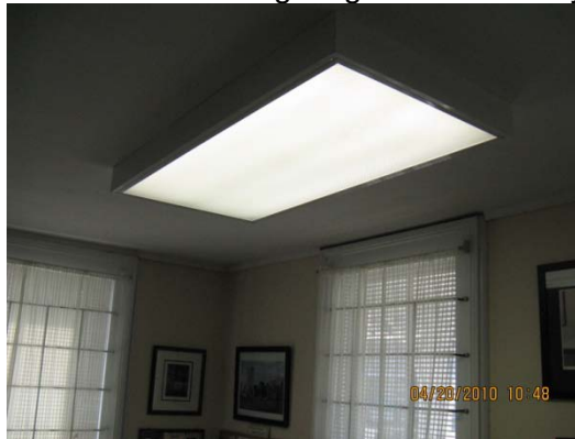
Typical Ceiling Mounted Fixture with T12 Magnetically Ballasted Bulbs
