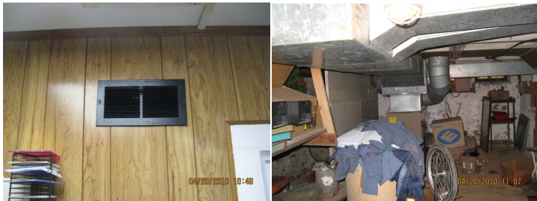
Examples of typical diffuser and distribution system in the basement
