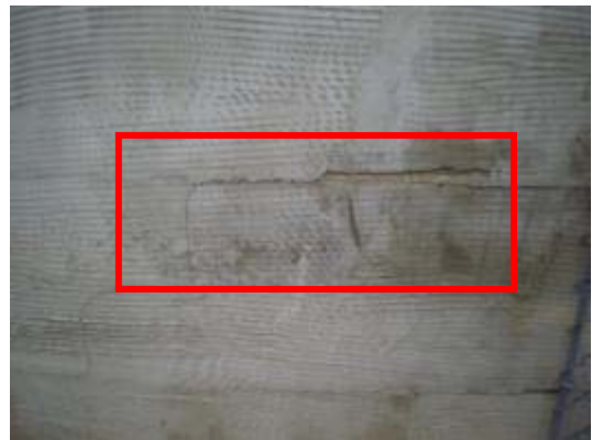
Damaged exterior wall finish with a damaged vinyl siding that exposes the interior wall to the elements and is a source of infiltration. Cracked concrete base and signs of water damage.
