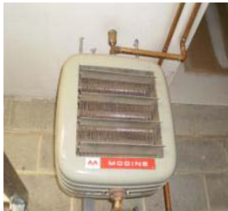
Modine unit heater in Garage
