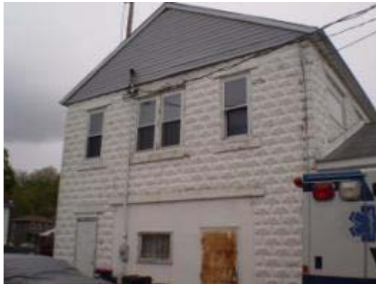
Damaged/aged window frame and air-leakage at sleeved window/wall air-conditioning units. Single-glazed window with ineffective frame
