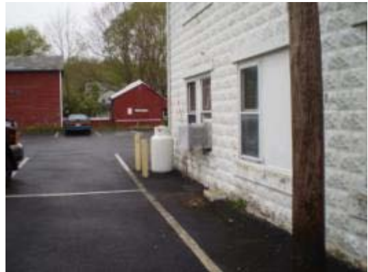
Damaged/aged window frame and air-leakage at sleeved window/wall air-conditioning units. Single-glazed window with ineffective frame
