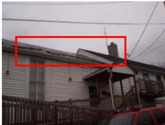
Sections of roof with damaged or displaced asphalt shingles and an improperly sealed cupola.
