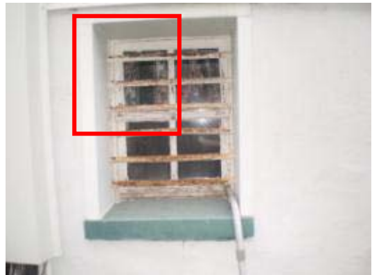
Damaged/aged window frame and single-glazed window with ineffective frame
