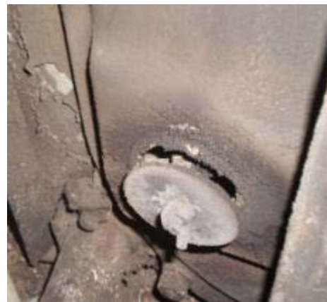
Weil-McLain boiler (L); Burner dislodge from boiler (R)
