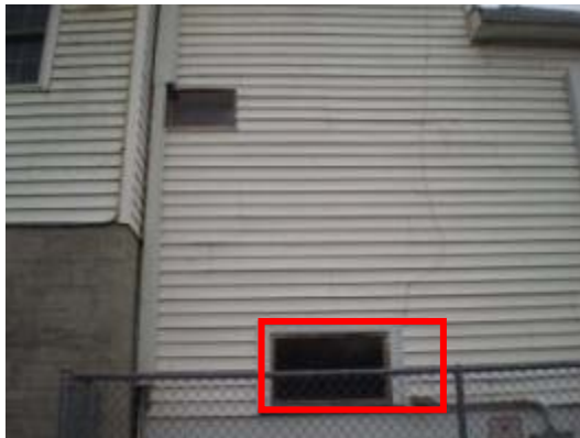
Damaged/aged window frame and single-glazed window with ineffective frame
