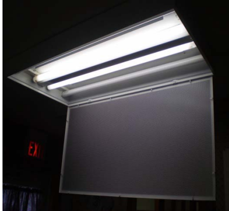
Typical Ceiling Mounted Fixture with T12 Magnetically Ballasted Bulbs
