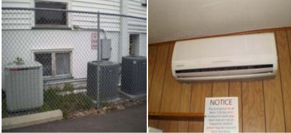
View of (3) Trane condensers (L); Typical Samsung evaporative unit in Library (R)
