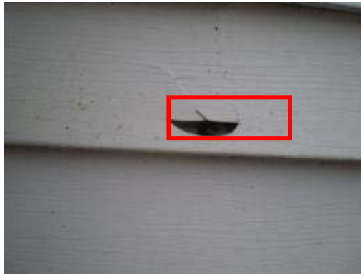
Damaged exterior wall finish with a damaged vinyl siding that exposes the interior wall to the elements and is a source of infiltration. Cracked concrete base and signs of water damage.
