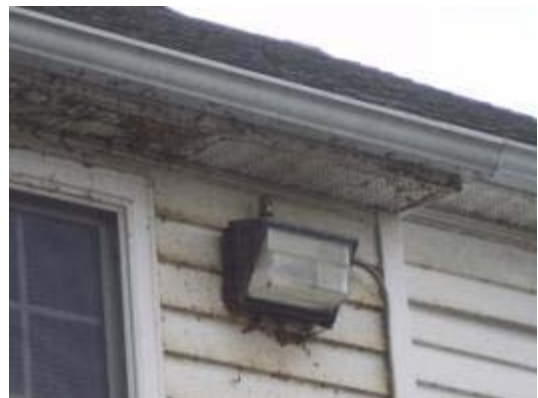
Damaged exterior walls with signs of water damage, sections with vegetation overgrowth and insect infestation.
