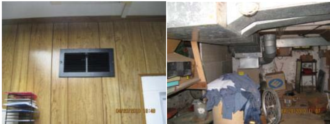
Examples of typical diffuser and distribution system in the basement
