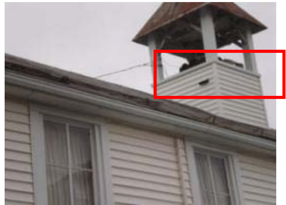
Sections of roof with damaged or displaced asphalt shingles and an improperly sealed cupola.
