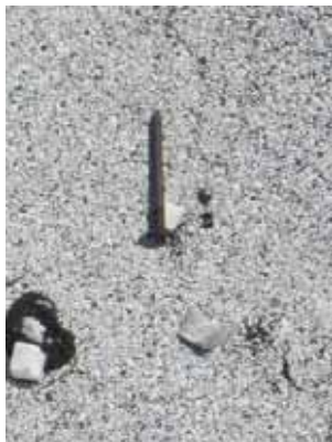
Rocks/nails or other sharp objects on roof surface
