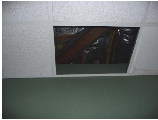
Missing ceiling tile by kitchen area; roof batt insulation is visible
