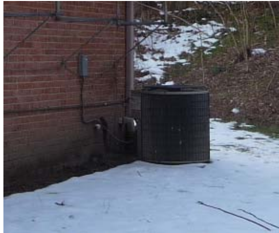
Payne Condenser, 3.5 Ton Capacity
