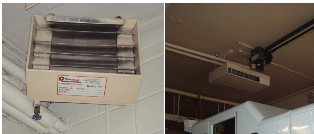
Hot water Unit Heaters in Truck Bay, Hot water heater (left); Cabinet Unit hot water heater (right)
