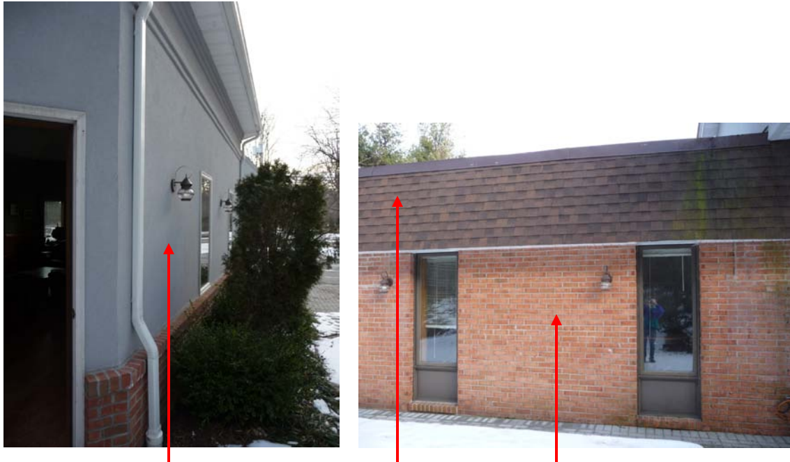
EIFS wall section and mansard above 4" brick veneer
