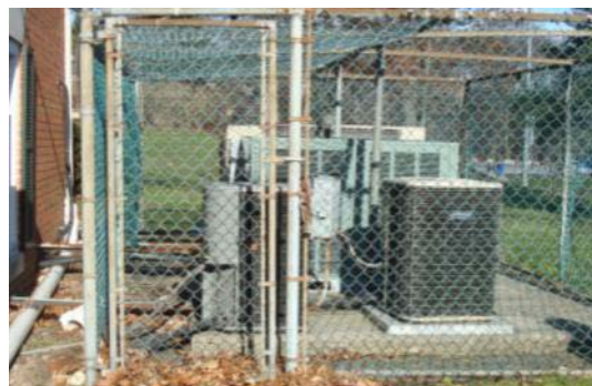
Condensers installed in back of Building
