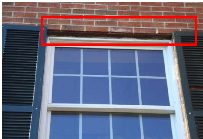
Window lintel needing caulking at the top as well as painting
