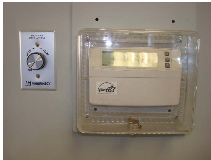
Greenheck exhaust variable speed control for exhaust fans (left) & Programmable thermostat for heaters (right)
