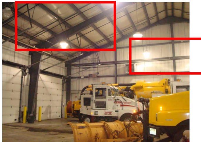
Roof / ceiling and wall batt insulation
