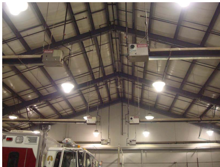
Main garage ceiling mounted heaters
