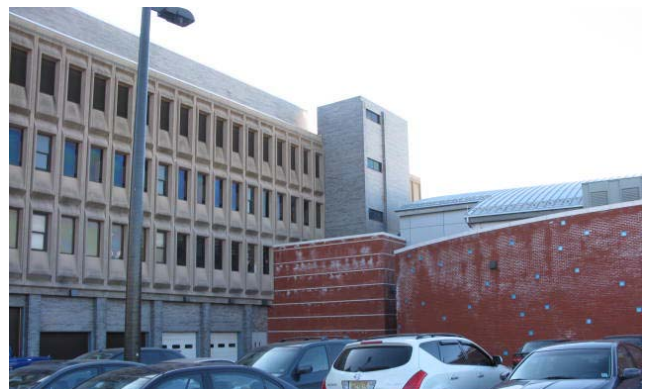
Efflorescence on Gym Walls
