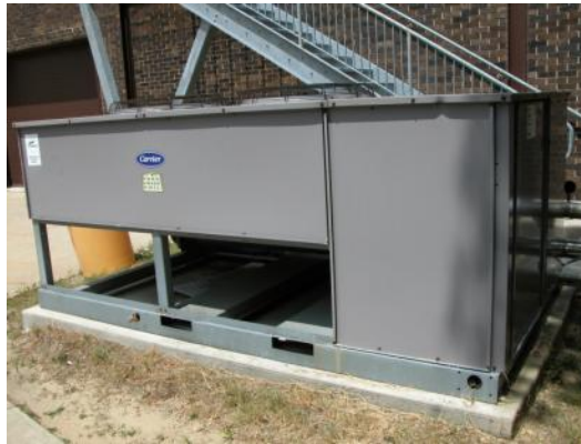
Carrier Air-Cooled Chiller
