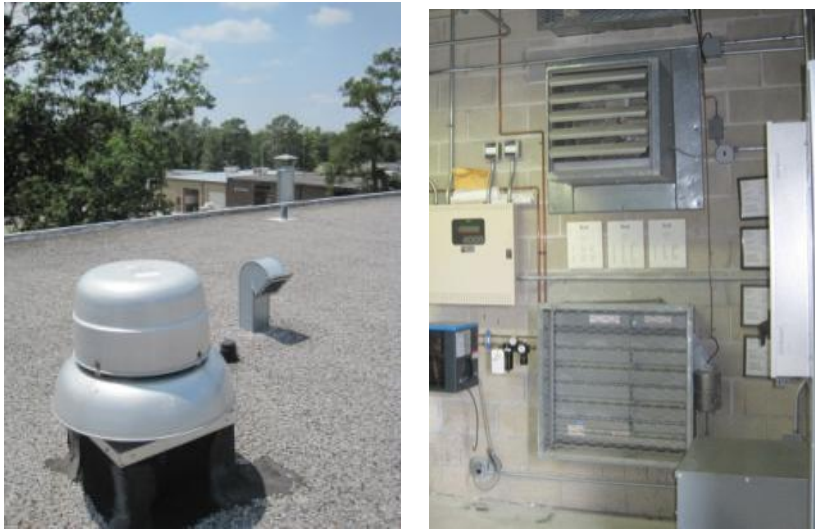
Rooftop Exhaust Fan; AHU-1 MER OA Intake Damper and Exhaust Fan
