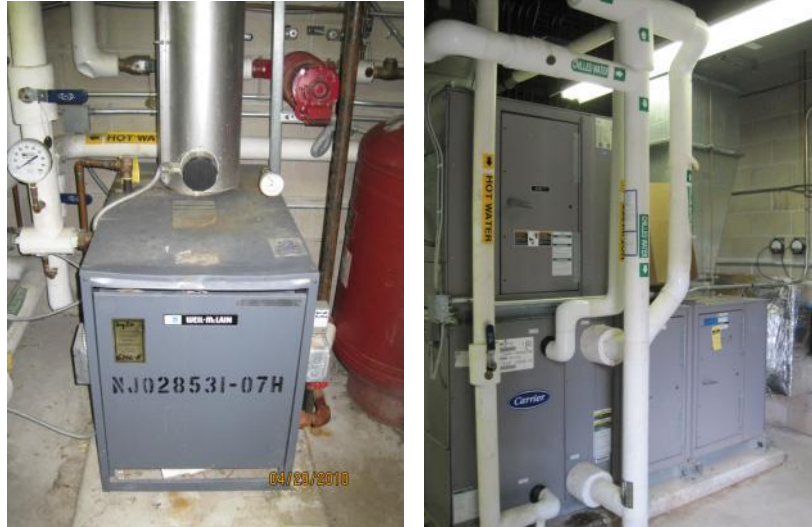
Stand-by Weil McLain NG Boiler; AHU-1
