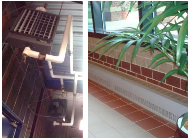
MER Penthouse HW Heaters; Fin Tube Radiators, Typ.
