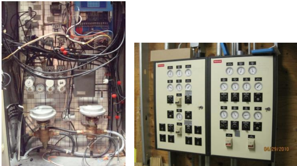
Pneumatic controller inside; outside
