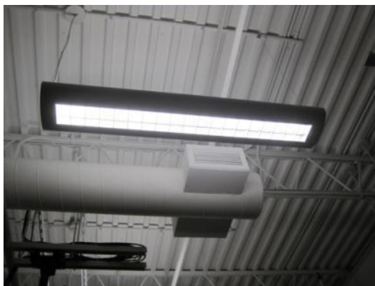
Ceiling Suspended T12 Fixture, Typ.; Lobby lighting
