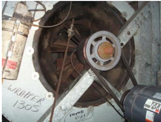
The AHU-1 supply fan damper blades inoperable
