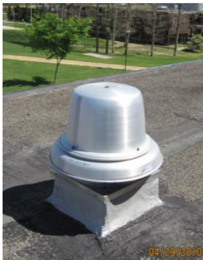
Rooftop Exhaust Fan, Typ., Outside Air Damper into MER Penthouse
