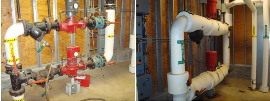
Hot Water Coil Booster Pumps; Chilled Water Coil Booster Pumps
