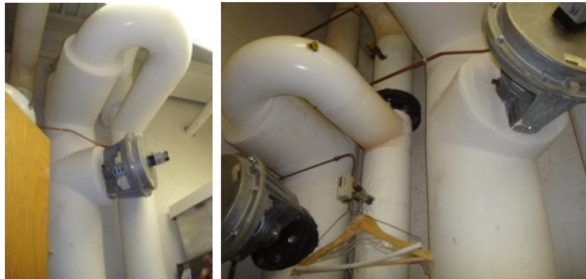
Hot Water and Chilled Water Supply and Return piping from/to the Central Plant with Pneumatic Valves
