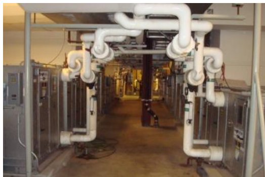
Air Handling Units in MER Penthouse with Heating and Cooling Coils
