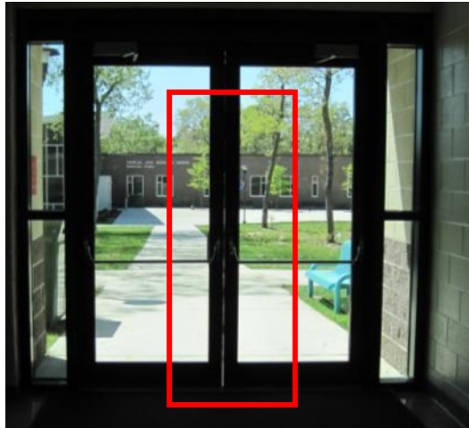
Missing/worn weather-stripping
