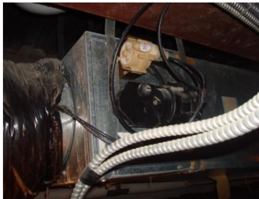
Variable Volume Box damper actuator, typ.
