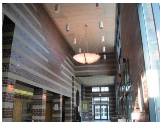
Ceiling Suspended T12 Fixture, Typ.; Lobby lighting
