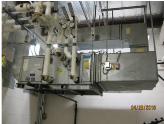
Suspended Air Handling Unit AHU-3 Serving Massage Area; New AHU-3 to replace existing
