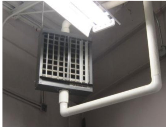
Cabinet Unit heater, typ.; Hot Water Unit Heater, typ.
