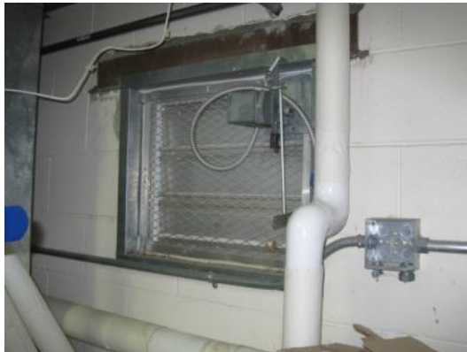
Pneumatic automatic outside air damper, typical; MER Return Fan, noisy
