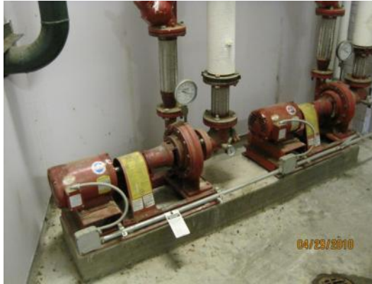
Primary Hot Water Pumps; Secondary Hot Water and Glycol Chilled Water Pumps
