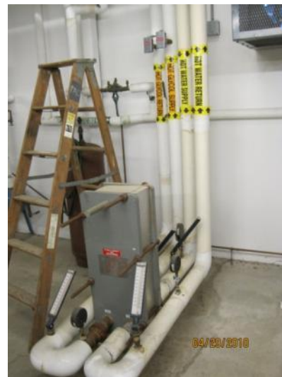
McQuay Air Cooled Glycol Chiller to be removed (Left); Hot Water to HW Glycol Heat Exchanger to be removed (Right)
