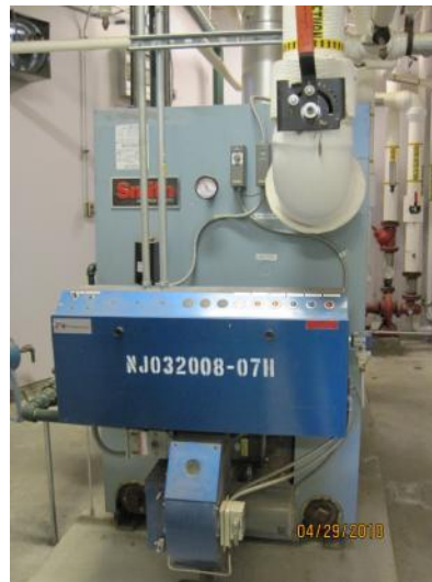
Smith Cast Iron Hot Water Boiler
