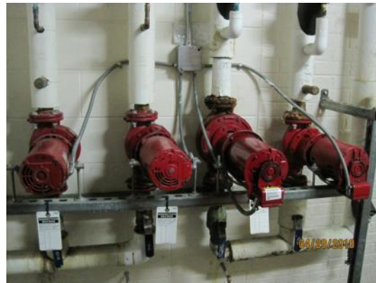
Primary Hot Water Pumps; Secondary Hot Water and Glycol Chilled Water Pumps
