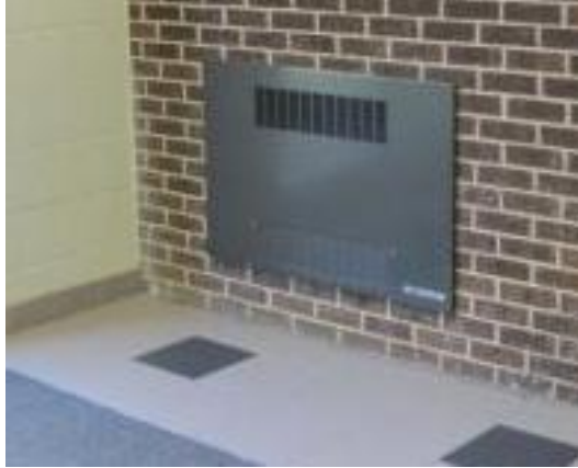
Cabinet Unit heater, typ.; Hot Water Unit Heater, typ.
