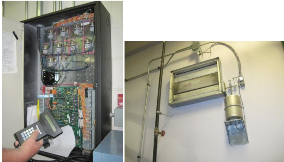
Electronic to pneumatic controller; Pneumatic piston, typ.
