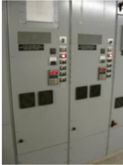
AHU-4 fan VFD Drives
