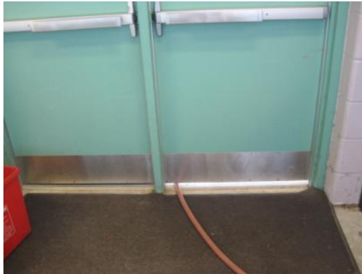
Missing/worn weather-stripping
