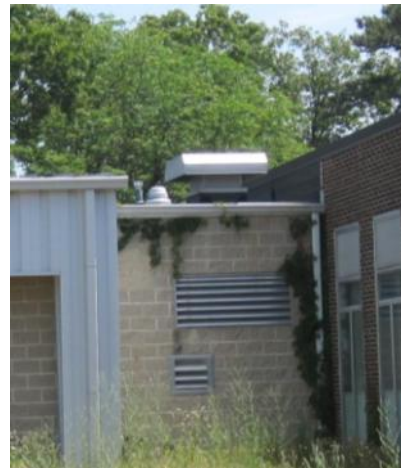
Overgrown ground vegetation blocking exterior wall surfaces which can damage exterior walls and contribute to moisture damage
