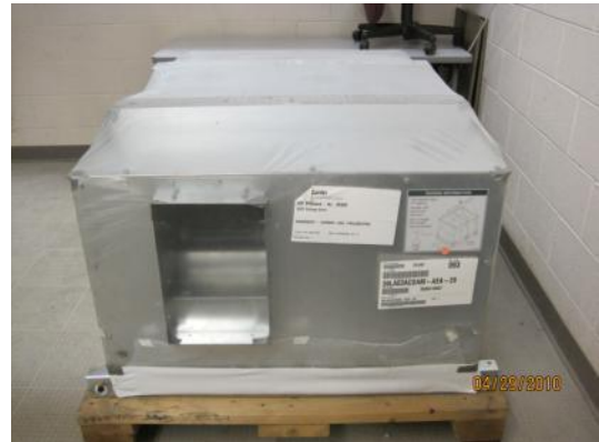
Suspended Air Handling Unit AHU-3 Serving Massage Area; New AHU-3 to replace existing
