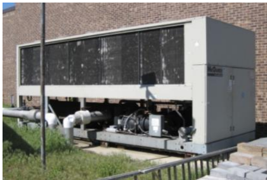
McQuay Air Cooled Glycol Chiller to be removed (Left); Hot Water to HW Glycol Heat Exchanger to be removed (Right)
