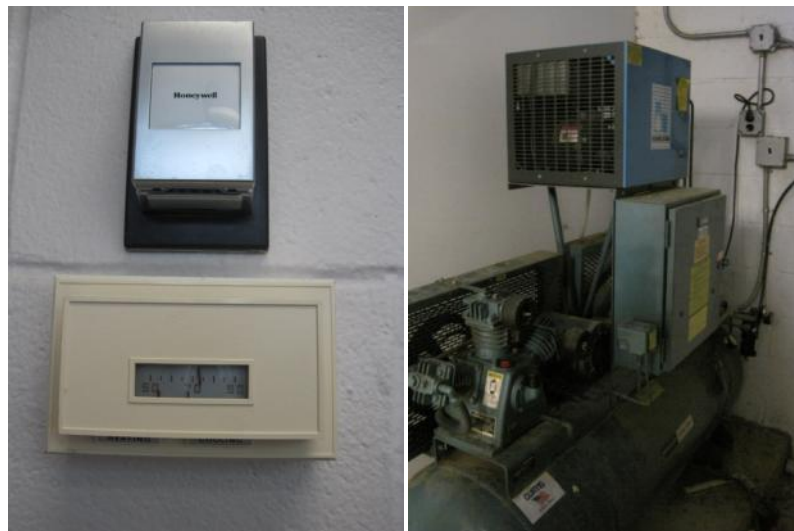
Thermostat and temp. sensor, typ.; Pneumatic Air Compressor & Air dryer
