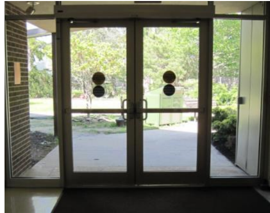
Missing/worn weather-stripping
