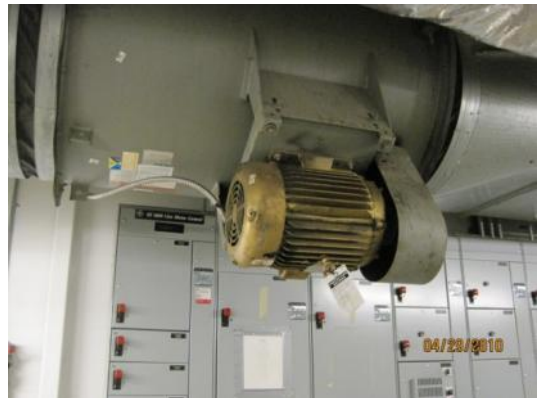
Pneumatic automatic outside air damper, typical; MER Return Fan, noisy
