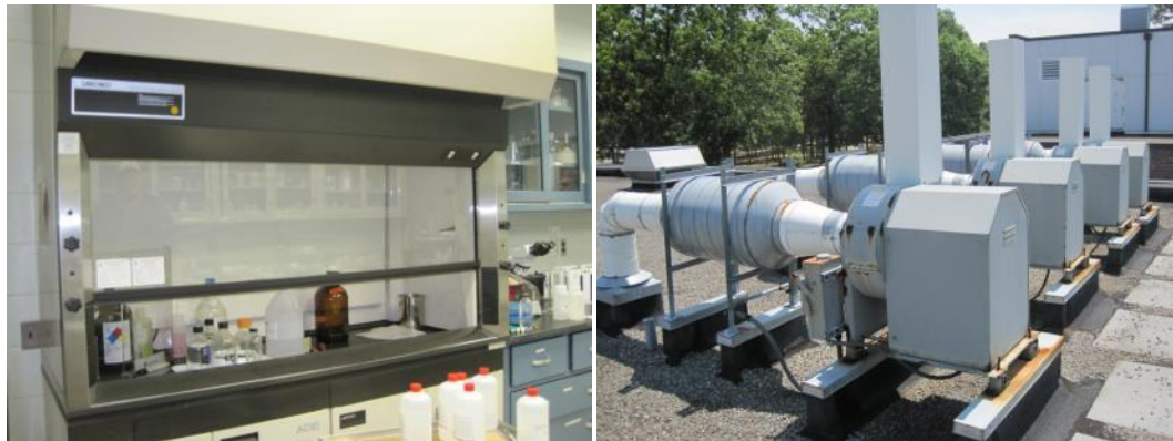
Laboratory Hood, typ.; Lab Hood Exhaust fan with sound attenuator, Typ.
