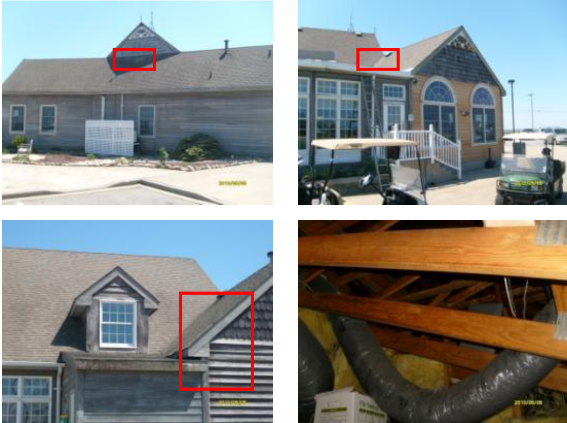
Examples of missing/ineffective flashing, damaged or displaced shingles, leaking/ineffective cap flashing seams, missing or damaged roof insulation.
