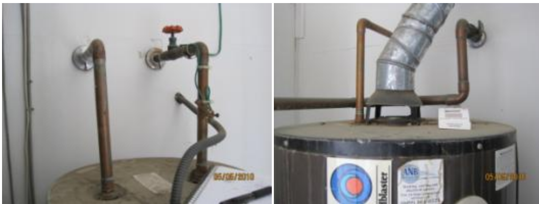
Un-insulated hot water piping
