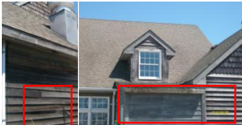
Examples of damaged and displaced wood siding and signs of mold and water damage
