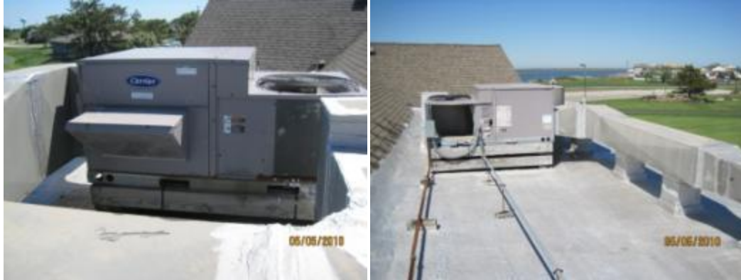
Front and Back View of Packaged Rooftop Unit
