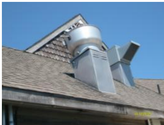
Rooftop exhaust fans serving the kitchen and dining room area
