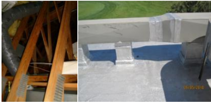
Air distribution system at the buildings exterior and attic
