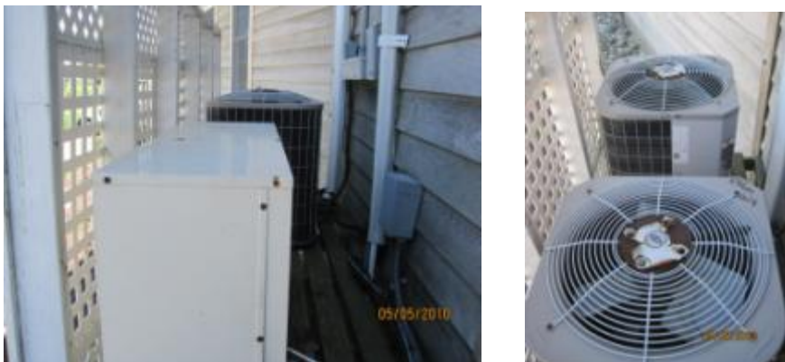
Typical condenser units installed at the clubhouse
