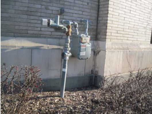
Existing gas meter and pressure regulator
