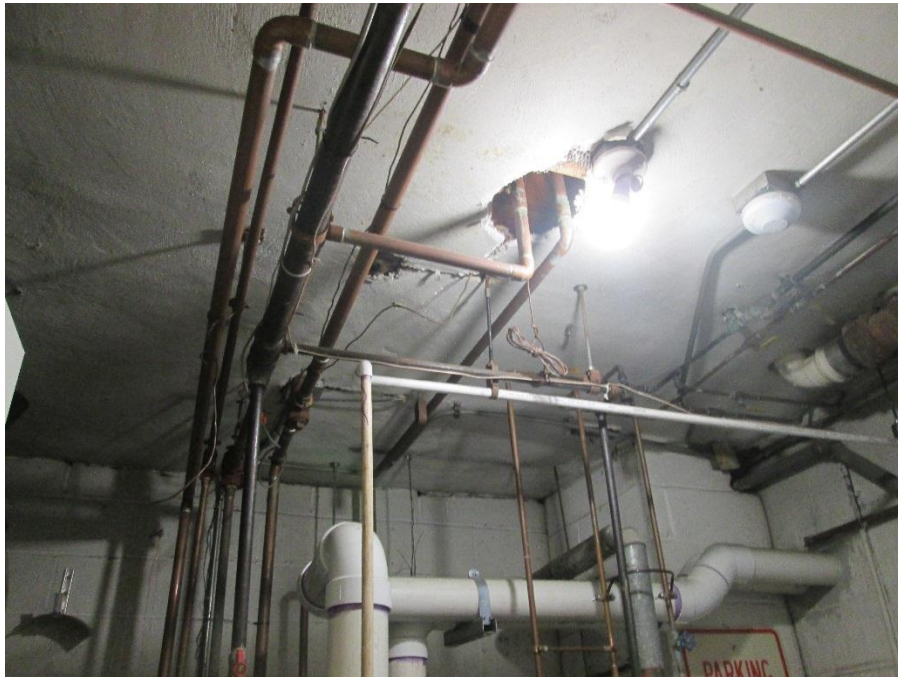
3. Existing Uninsulated Piping in Boiler Room
