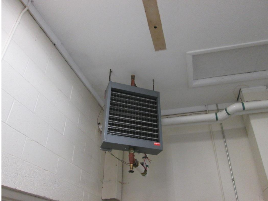
1. Hot Water Unit Heater
