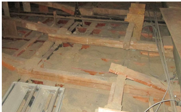
2: Existing attic insulation
