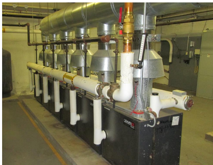
2: One row of six Caravan Slant Fin hot water boilers
