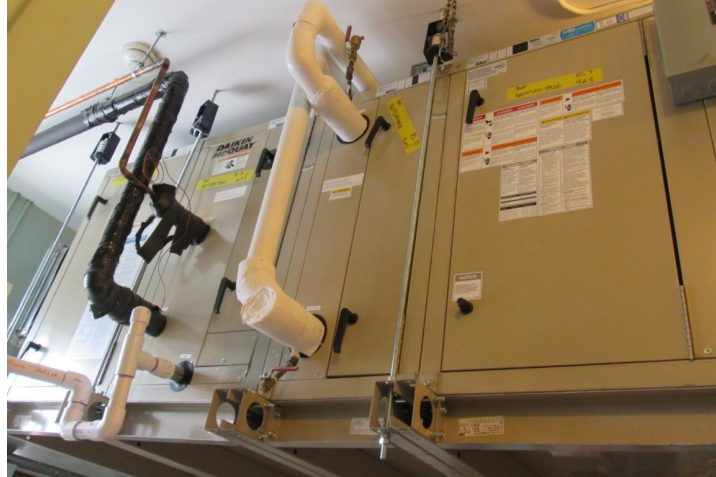
3: New Daikin McQuay AHU for Multi-purpose room
