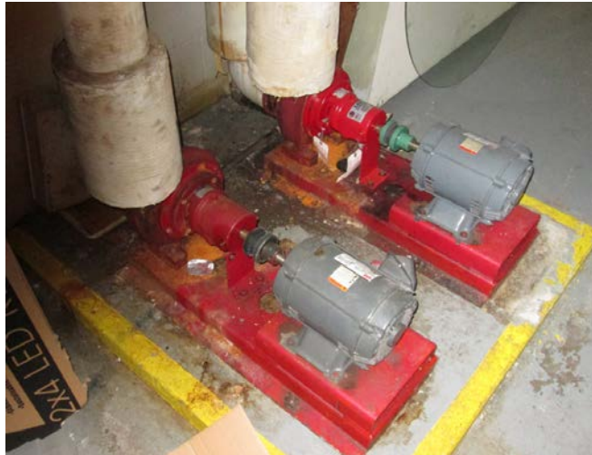
5: Base mounted system pumps w/o VFDs
