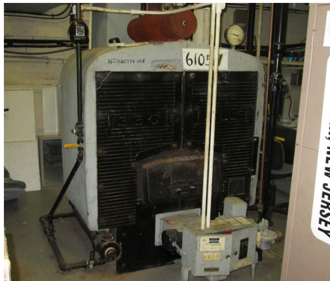
2: H.B. Smith 1968 hot water boiler
