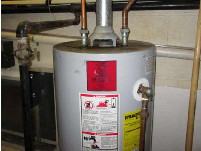
4: Existing domestic hot water heater
