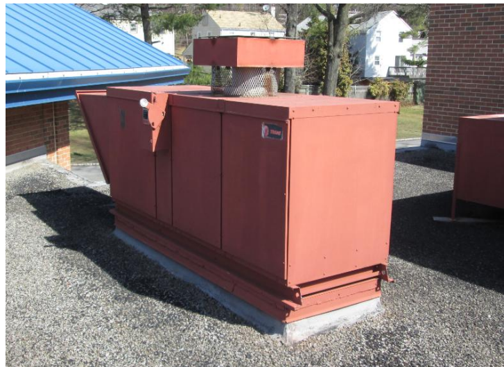
2: Trane rooftop unit vintage 1996
