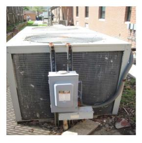
ECM-4 Replace Chiller serving the North wing with a High efficiency chiller
