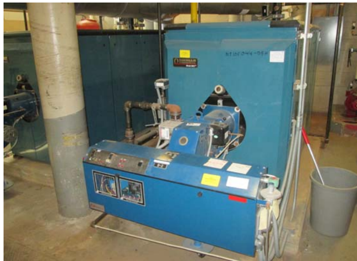
2: Burnham cast iron sectional boilers
