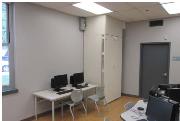
2: Aerdaale heating, cooling, & ventilating unit
