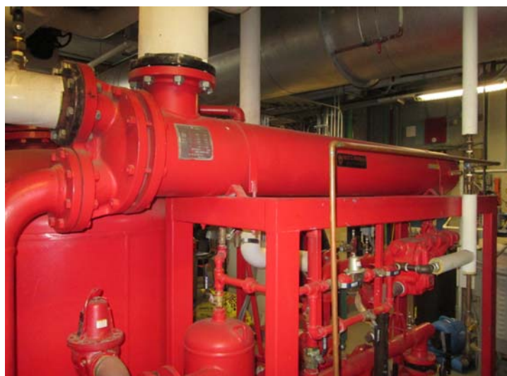
2: Steam-to-hot water generator
