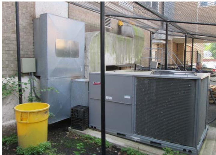
5: Kitchen MAU unit and associated ductwork
