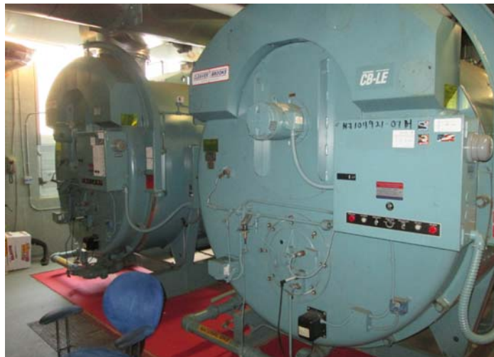
2: Cleaver Brooks steam boilers
