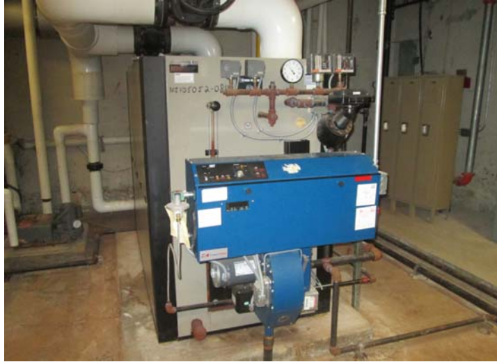
4: Gas fired steam boiler
