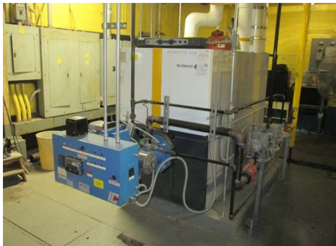
2: One of two De Dietrich hot water boilers
