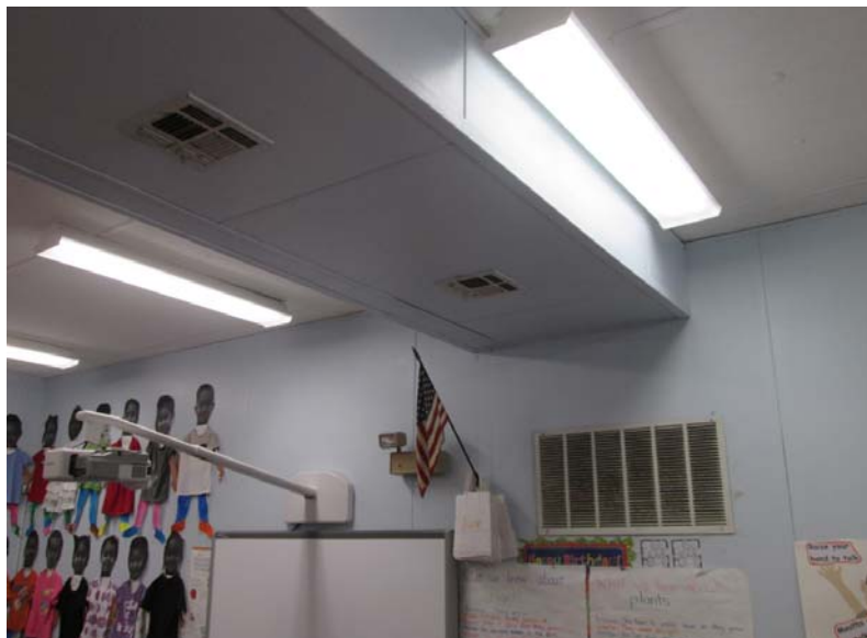
5: Modular classroom—HVAC supply and return air grilles
