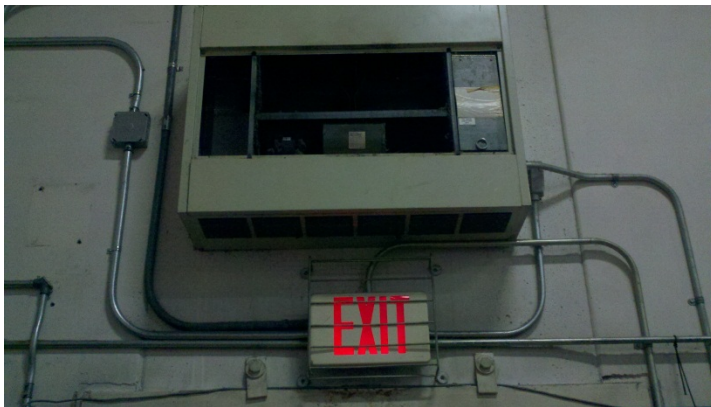
Figure 5 Electric Cabinet Heater in GYM(Missing Cover)
