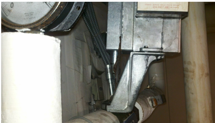
Figure 3 Disconnected Control Valve
