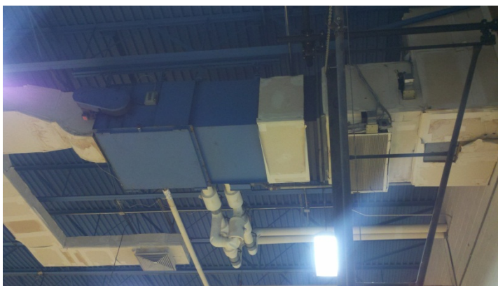
Figure 6 Air Handling Unit In GYM
