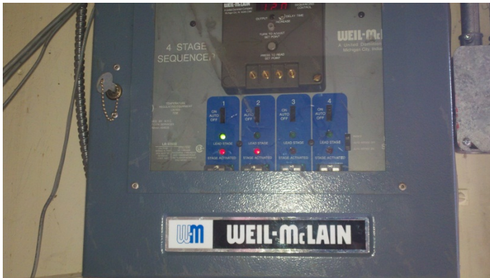
Figure 2 Boiler Control Panel (Non Operational)
