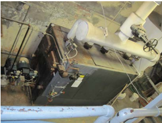
2: Typical steam boiler
