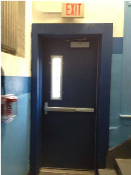
1: Existing door seals
