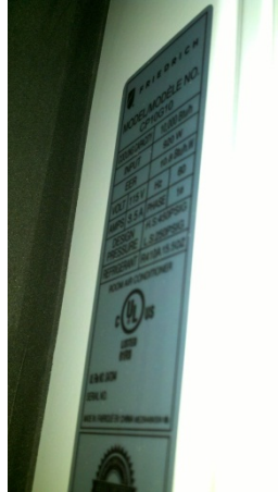
1: Sample window A/C nameplate
