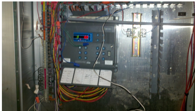
3: Johnson HVAC Controls System
