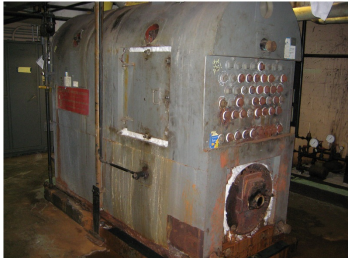
2: Existing HHW boiler
