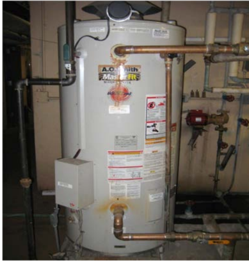
4: Existing Hot Water Heater
