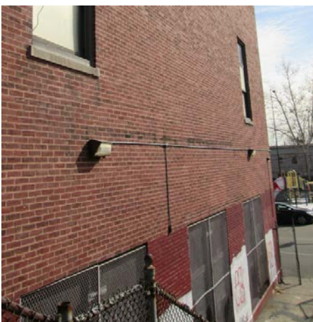
6: Rear exterior wall with wall-pack lighting
