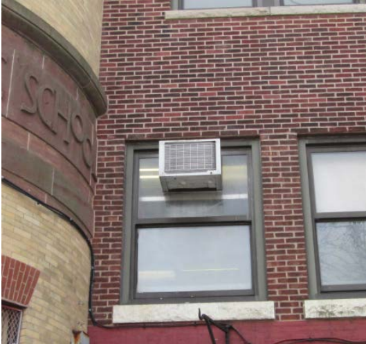
4: Franklin school with window air conditioning unit
