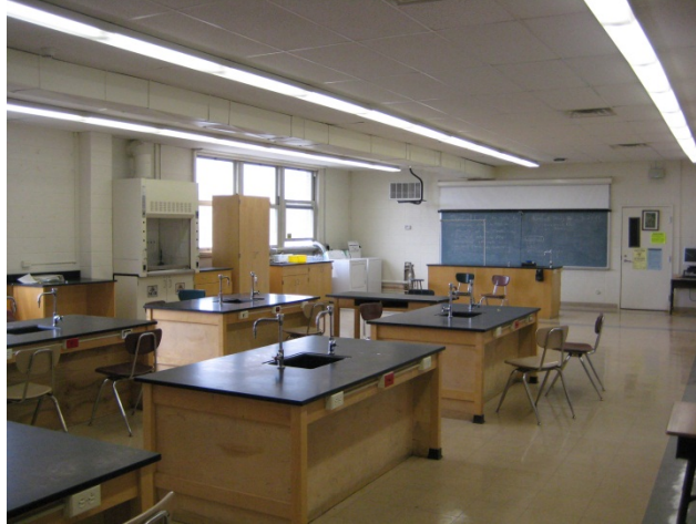
9: Sample classroom lighting fixtures
