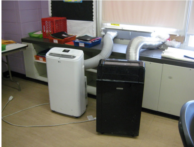
3: Portable window air conditioning unit
