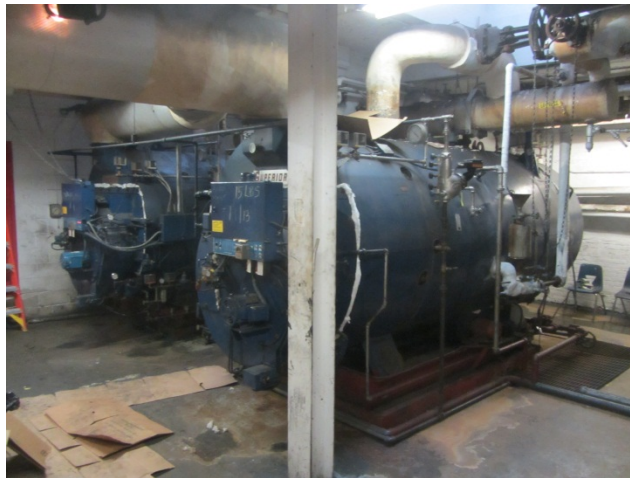
2: Existing oil fired boilers
