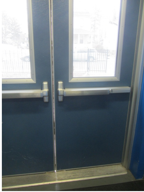
1: FRP doors with bad seals; gaps visible which allow outdoor air infiltration
