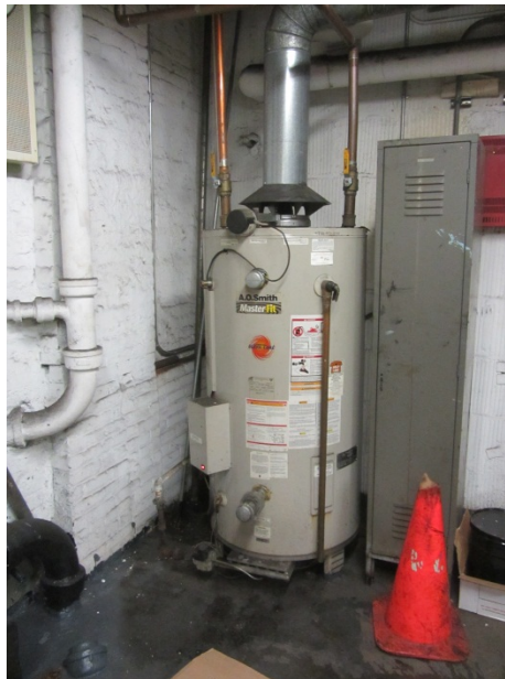
4: Existing natural gas fired DHW heater
