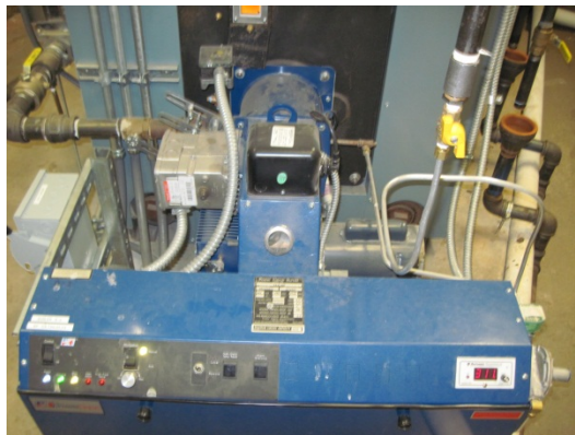
3: Existing Burner for Steam Boiler
