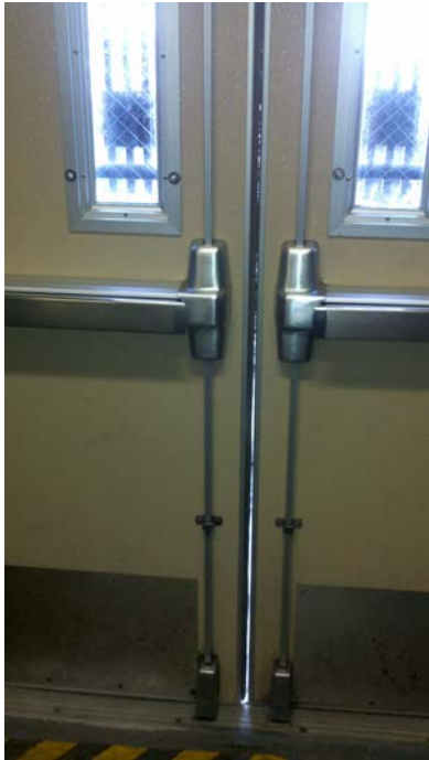
1: Gap allows excess infiltration
