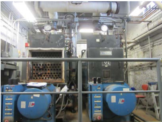
2: Steam systems operate less efficiently than HW
