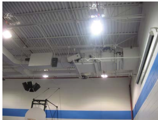
5: Existing Gym Unit. Existing Metal Halides in Gym also.
