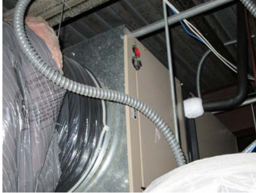
1: Existing Split System above Office w/ Electric Heat
