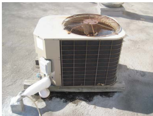
3: Existing Condensing Unit for Office Unit. Located on Roof
