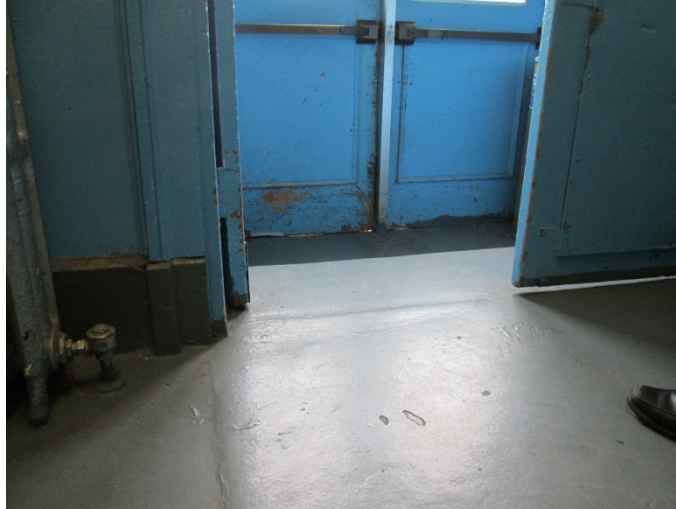
1: Deteriorated door sweeps allow excessive infiltration
