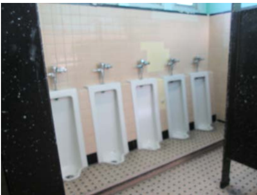
6: High flow plumbing fixtures
