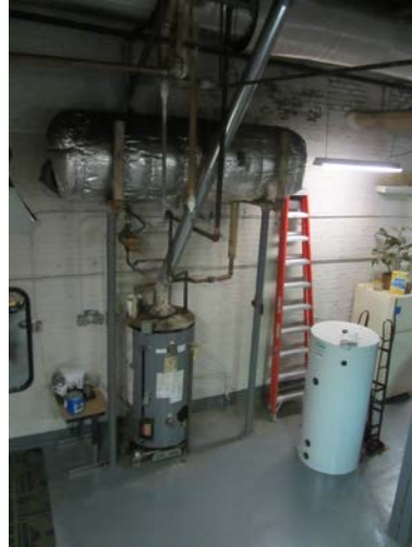
3: Picture depicting uninsulated DHW piping
