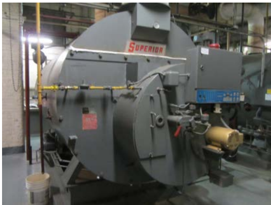
2: One of two oil fired steam boilers in boiler room
