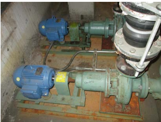
3: Existing HHW pumps and motors
