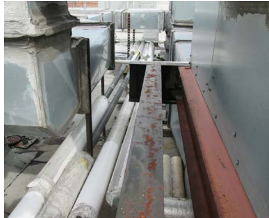
5: Un-insulated piping on roof
