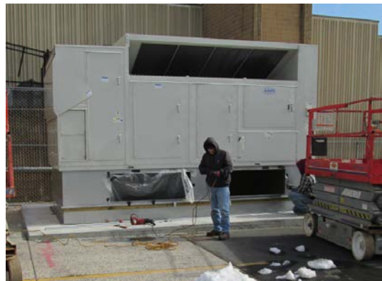
5: New ERU being installed on outdoor concrete pad
