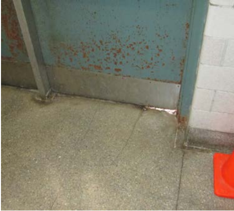
1: Daylight visible beneath exterior door
