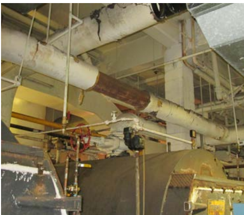
3: Degraded insulation on existing steam piping
