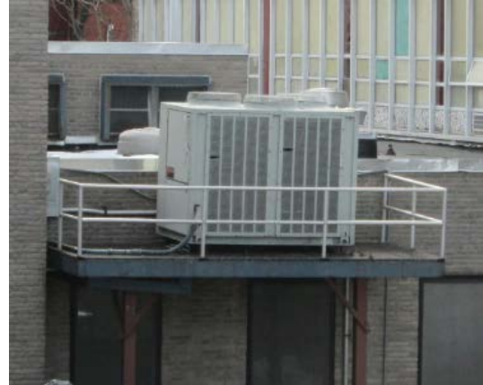
4: Trane air-cooled condensing unit
