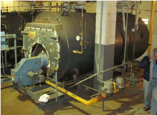
2: Titusville firetube boiler should be replaced
