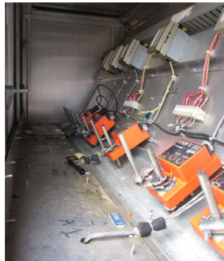
6: Temperature zone controllers for AC-2 RTU
