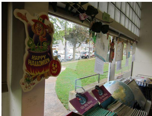
Non-insulated metal frame with single-glazing provides poor insulation to the building
