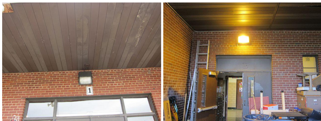
Typical wall pack high pressure sodium fixtures
