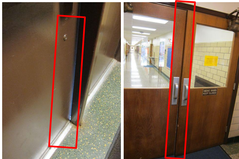
Exterior door at the southeast end lacks weather-stripping (R) and vestibule doors can no longer be shut completely (L)
