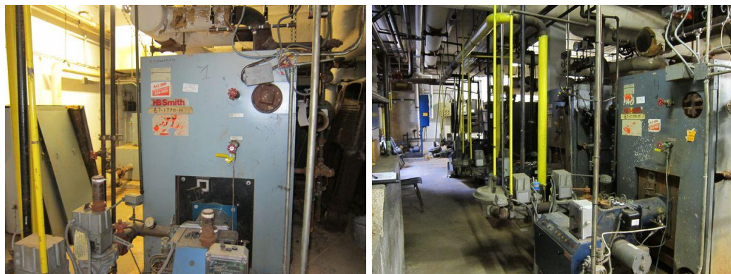
HB Smith steam boiler (R) and Aerco hot water boilers (L)
