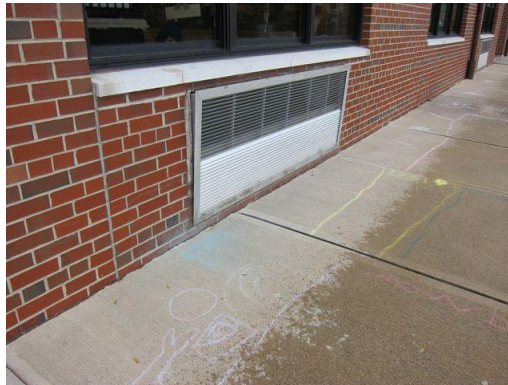
Poorly installed unit ventilator grill compromises building air-tightness
