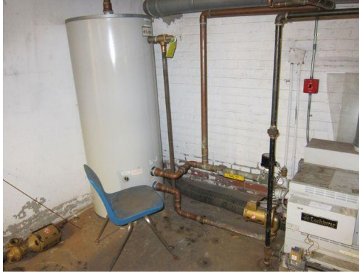
Gas-fired domestic hot water heater with storage tank. Note: all pipes for this system lacked proper insulation
