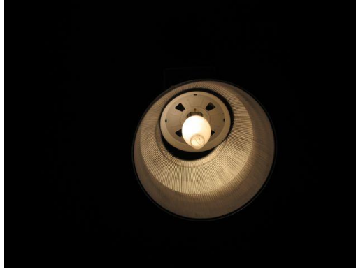
Typical high bay high pressure sodium fixture
