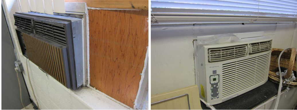
Typical window mounted AC units, permanently installed
