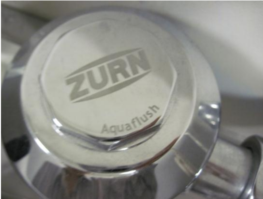
Existing Plumbing Fixtures
