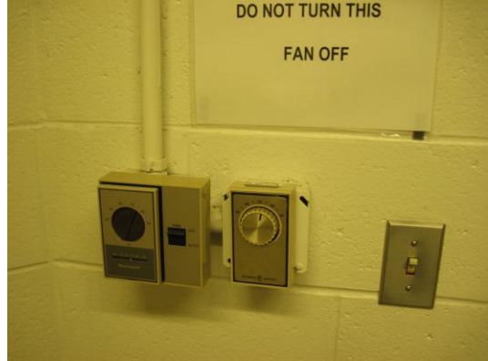
Manual Light Switches
