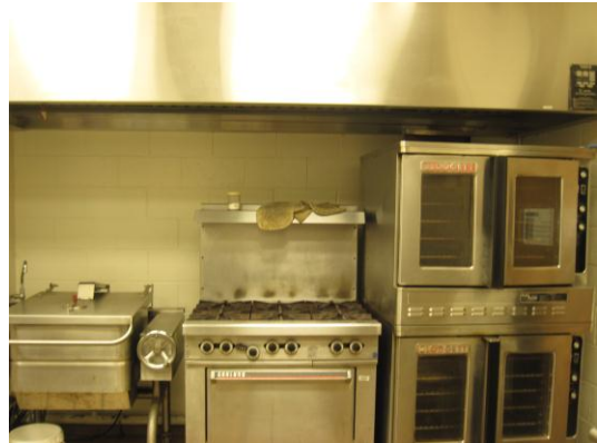
Existing Kitchen Hood
