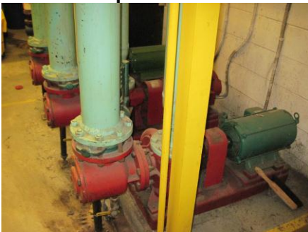
Existing Water Loop Pumps
