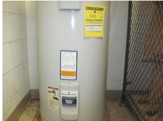
Existing Electric Water Heater
