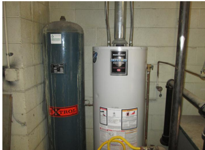
5: DHW heater and adjacent storage tank
