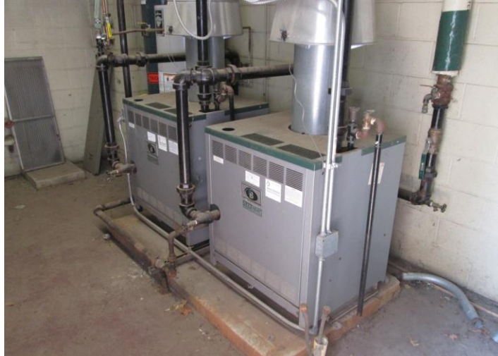
4: (2) hot water boilers that serve the building
