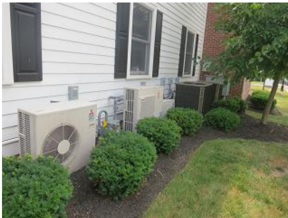
Image 5: Outdoor Condensing Units
