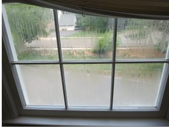
Image 4: Double pane vinyl window showing signs of breaks in seal.
