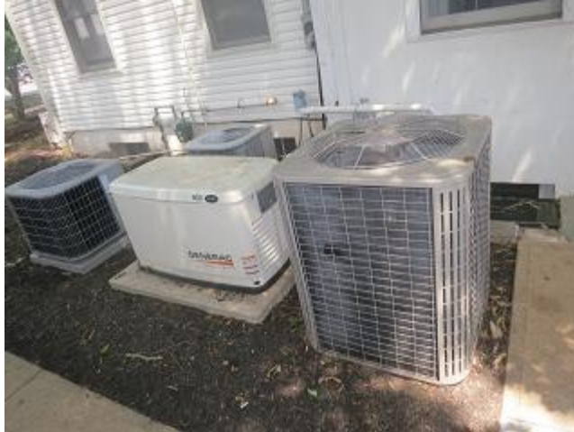
Image 7: Outdoor Condensing Units
