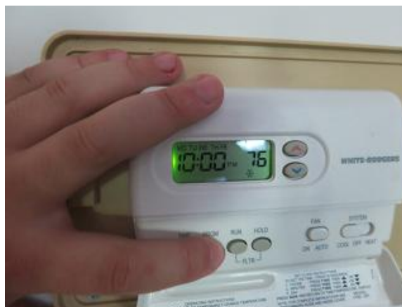
Image 9: Thermostat maintaining 76°F during unoccupied times
