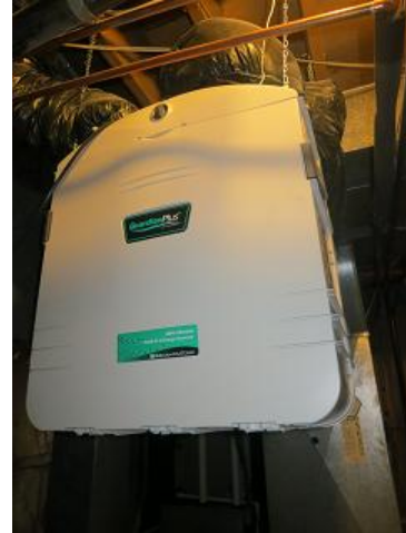
Image 8: Energy Recovery Ventilator
